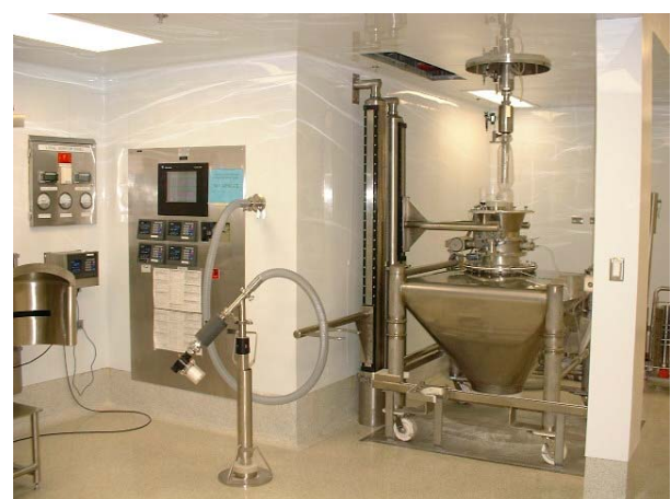
IBC Fill Station
